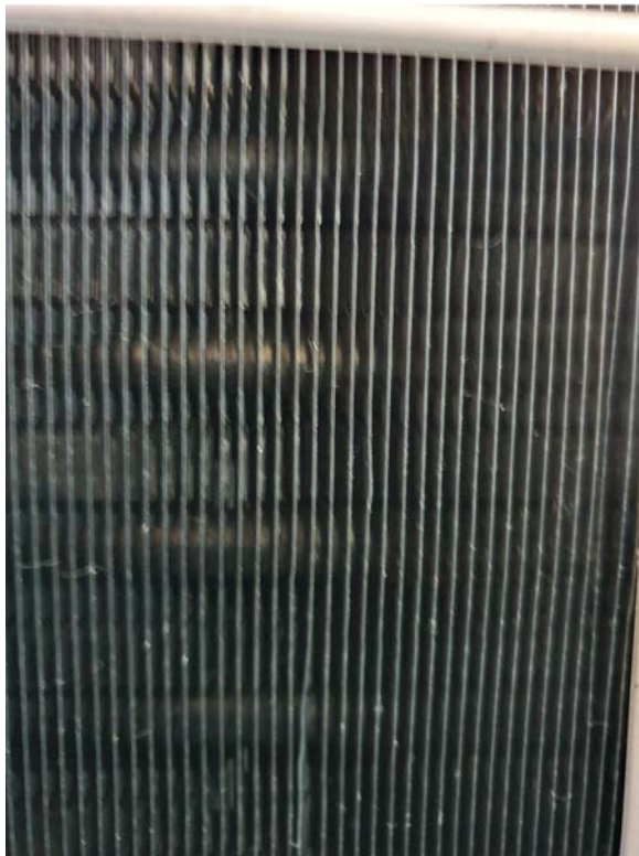
Figure 2 The Condenser after cleaning and treatment
